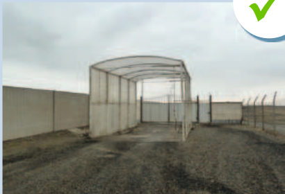
Disinfection tunnel for vehicles
