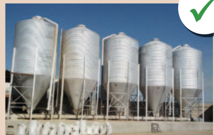
Silos in good conditions
