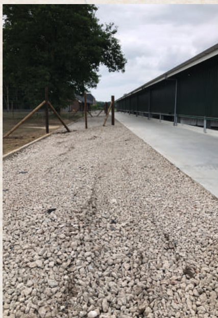
Clean, concrete, stones, tree roots for entrance barn or wintergarden
