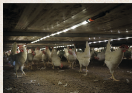
LED light to prevent floor eggs under the system
