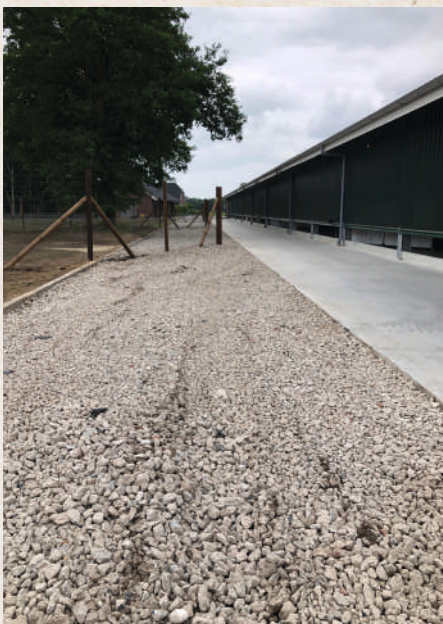
Clean, concrete, stones, tree roots for entrance barn or covered porch
