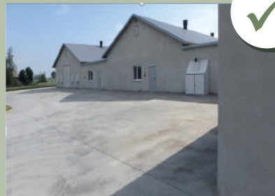
Surrounding concrete zone
