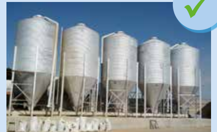
Silos in good conditions
