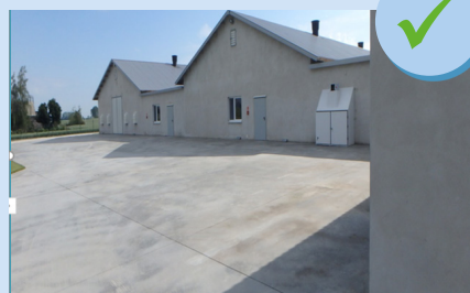
Surrounding concrete zone
