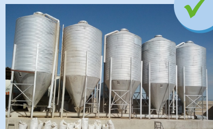
Silos in good conditions
