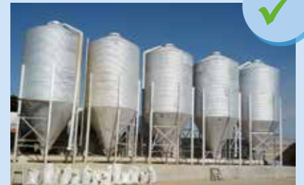
Silos in good conditions
