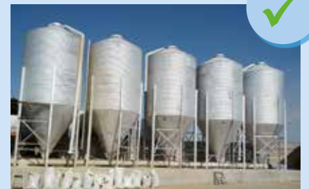
Silos in good conditions
