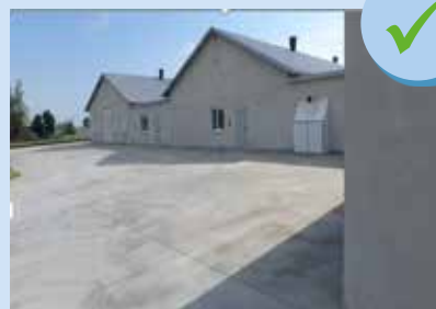
Surrounding concrete zone
