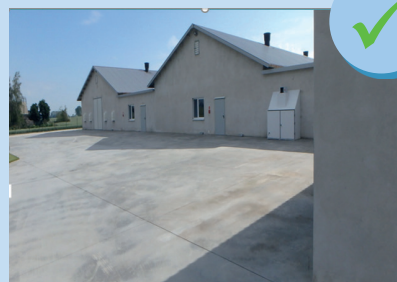
Surrounding concrete zone
