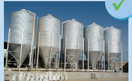
Silos in good conditions
