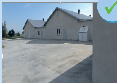
Surrounding concrete zone
