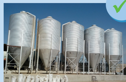
Silos in good conditions
