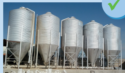
Silos in good conditions
