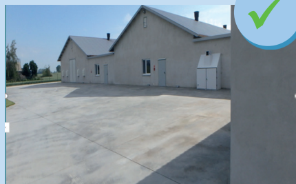
Surrounding concrete zone
