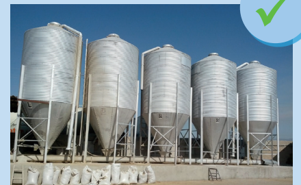
Silos in good conditions
