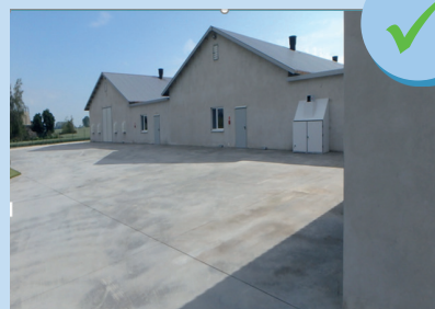
Surrounding concrete zone
