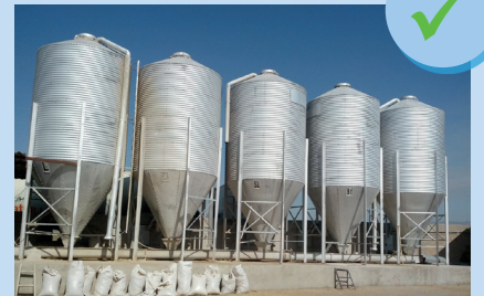
Silos in good conditions
