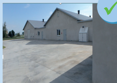
Surrounding concrete zone
