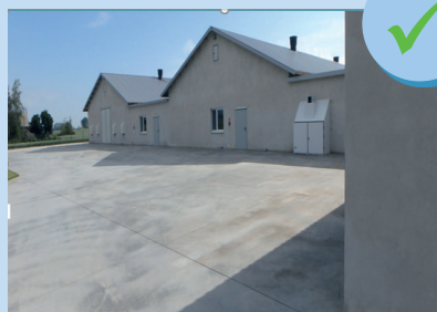
Surrounding concrete zone
