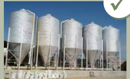
Silos in good conditions
