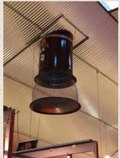
Under pressure climate control system in free-range barn
