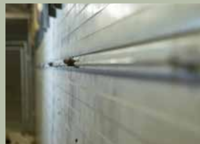
Fog installation in rearing house
