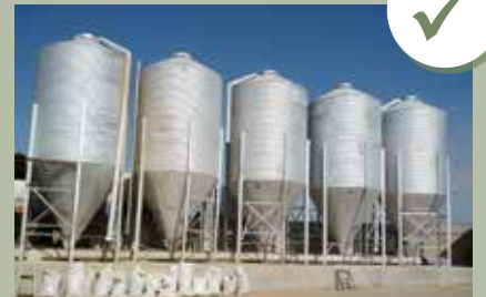
Silos in good conditions
