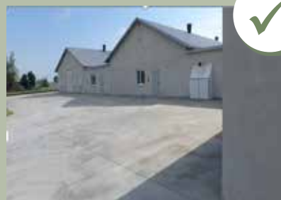
Surrounding concrete zone
