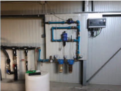
Water chlorination station
