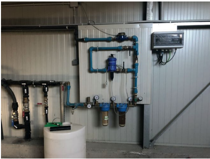
Water chlorination station
