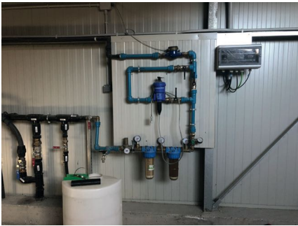
Water chlorination station
