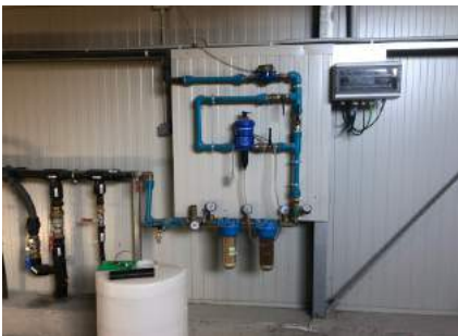
Water chlorination station
