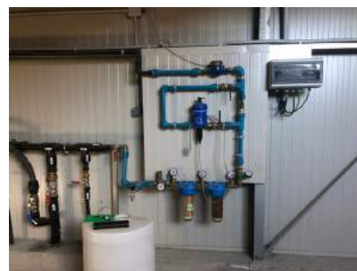
Water chlorination station
